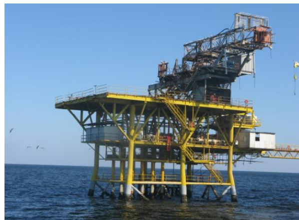
Figure 1. Nosrat Jacket Platform [48]
