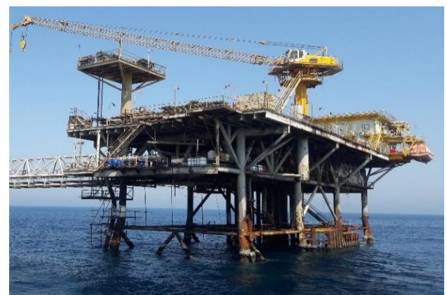
Figure 1. General View of the Drilling Platform
