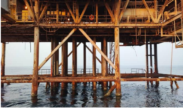
Figure 2. General Condition of Members in Splash zone
