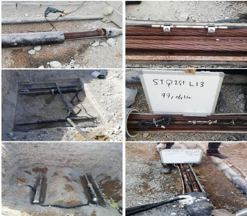
Figure 7. Installation steps of fiber optic strain gauge
