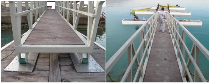
Fig. 3. A view of the access bridge to the composite floating dock
