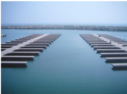
Fig. 1. Example of Floating Dock and Parking Structures for Mooring
