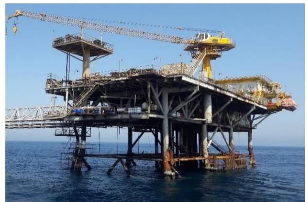
Figure 1. General View of the Drilling Platform
