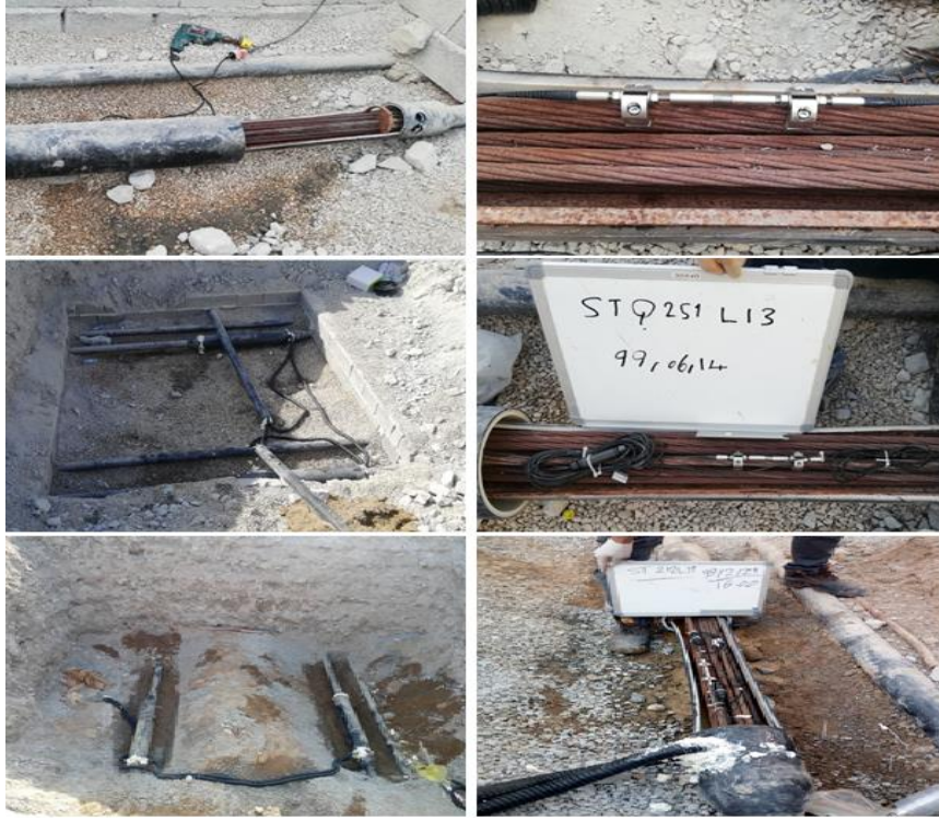
Figure 7. Installation steps of fiber optic strain gauge
