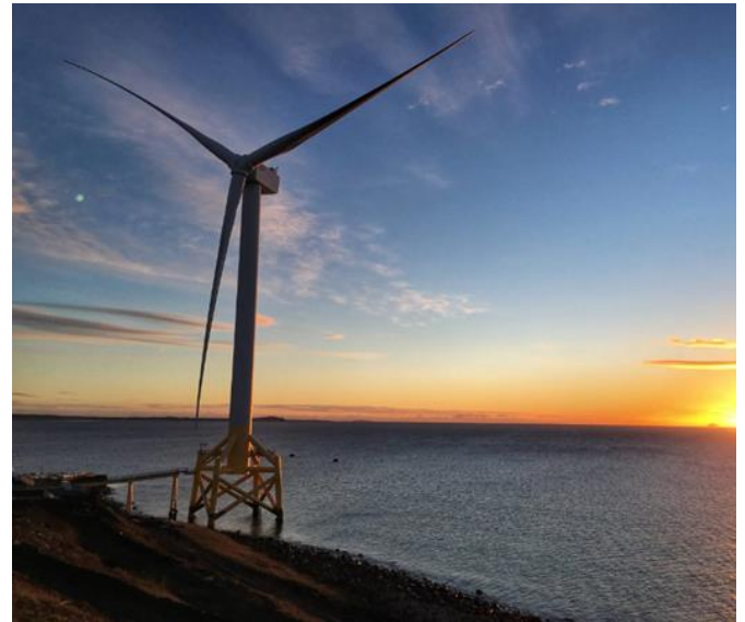
Figure 1. Levenmouth 7MW offshore wind demonstration turbine
