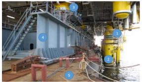
Figure 1 Floatover hardware [7] – (1) Stabbing Cone (2) Leg Mating Units inside jacket legs with receptor cone (3) Deck Support Unit (4) Deck Support Frame (5) Barge
