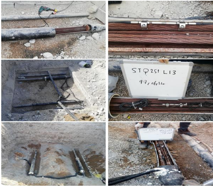
Figure 7. Installation steps of fiber optic strain gauge
